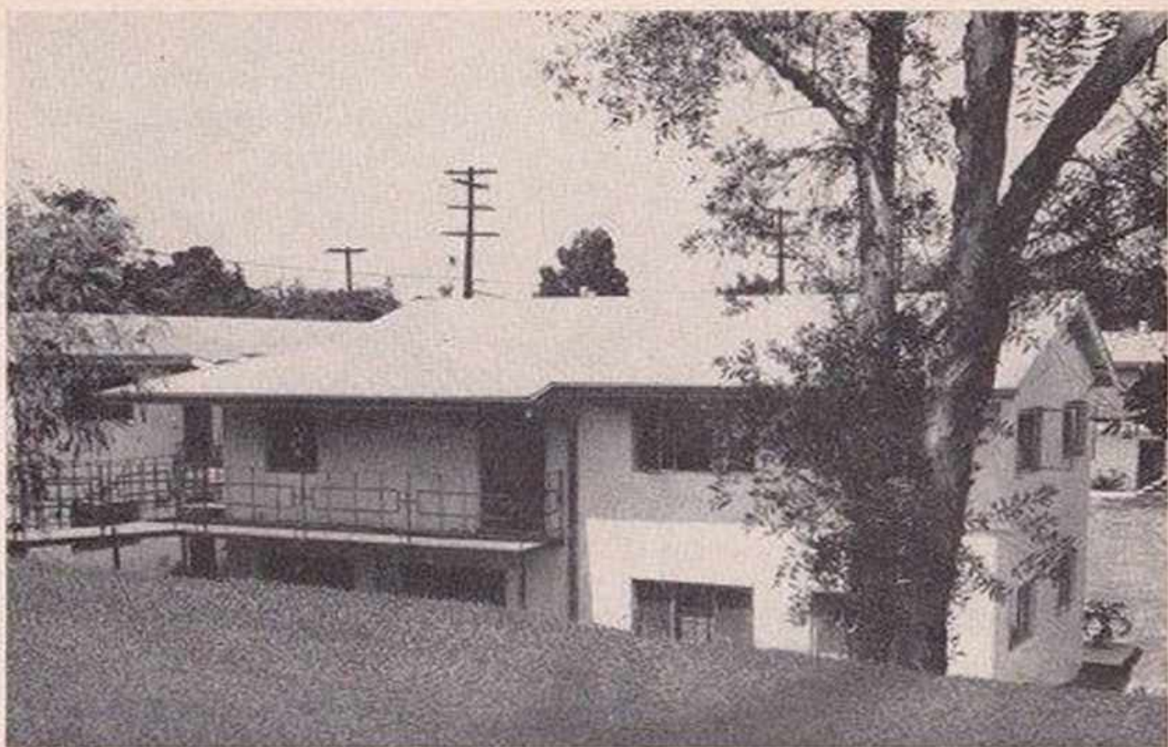
Rear of new refectory building for SRF monks, Los Angeles headquarters
